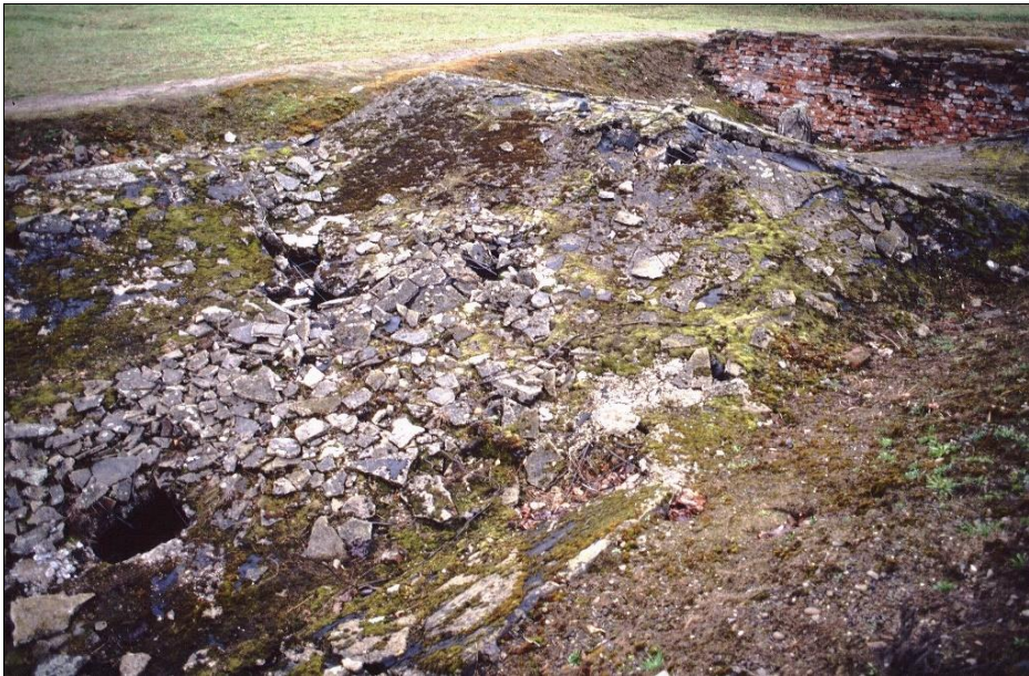
Figure 64: Morgue #1 of Crematorium II in Birkenau, collapsed roof, somewhat intact rear section. Left: square-shaped hole chiseled through the roof after its destruction, with reinforcement bars merely bent back (see Figure 86, p. 142). (February 1997)
