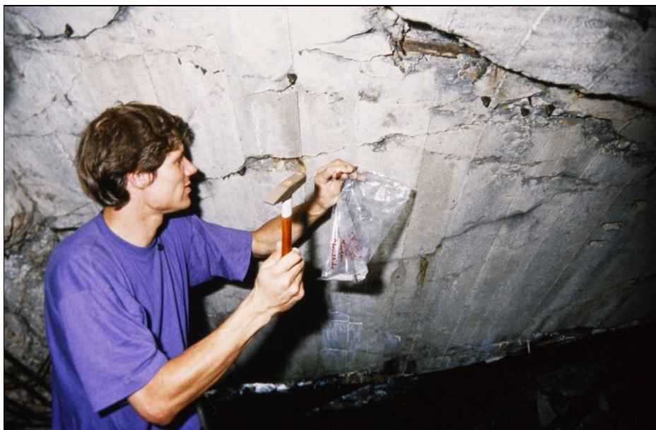
Figure 85: Ceiling of Morgue #1 (“gas chamber”) of Crematorium II with the author in August 1991. Sampling location of Samples 1 and 2.
