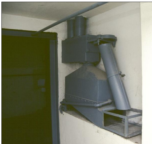
Figure 33: Look inside a Degesch circulation delousing chamber at the former Dachau Camp. (1998)
