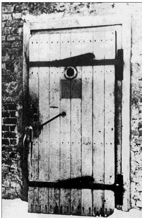
Figure 133: Wooden makeshift "gastight" door of the delousing gas chamber in the personal-effects storage area "Kanada I," 2 m × 1 m, with the upper end of the peephole at a height of some 1.60m; manufactured by the Deutsche Ausrüstungswerke (Pressac 1989, p. 46).
