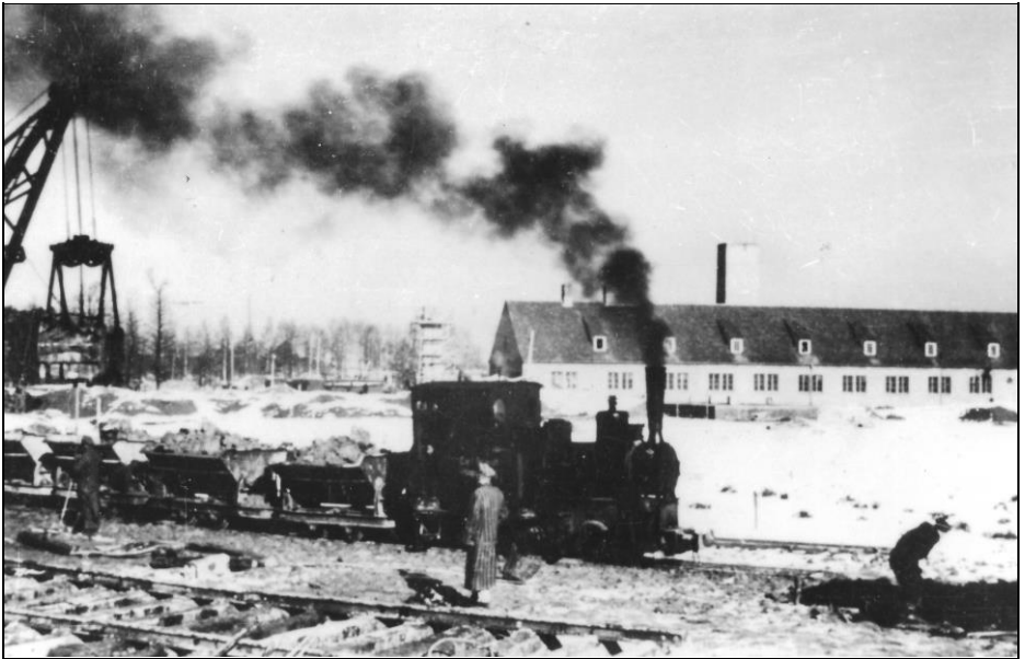
Figure 76: Photograph of Crematorium II of Birkenau taken in early February 1943 (Czech 1989, p. 454; Pressac 1989, p. 340).
