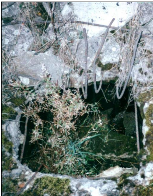
Figure 86: Hole in the roof of Morgue #1 (“gas chamber”) of Crematorium II in December 1991. It is clearly visible that it was not cleared of the steel reinforcement rods. These were simply bent back. © Carlo Mattoigno
