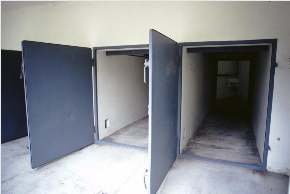
Figure 74: Gastight, escape-proof steel doors to the Degesch circulation delousing chambers at the Dachau Camp. (1998)
