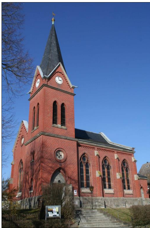
Figure 8: In August 1976, the Protestant church at D-96484 Meeder-Wiesenfeld was fumigated with Zyklon B. Subsequently, blue-colored stains appeared all over the plaster (see Figure 9).
