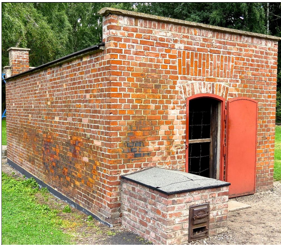
Figure 125: Zyklon-B-disinfection chamber in Stutthof Camp, south side, exterior. (© Jeff Linamen 2013)
