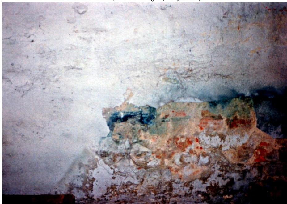
Figures 150a&b: Interior of the disinfestation wing of Building BW 5b, western part of the southern wall. The plaster, rich in lime, is only slightly stained. It has fallen off in certain areas. The mortar underneath is much more stained, see the close-up photo below. (© C. Mattogno, July 1992)
