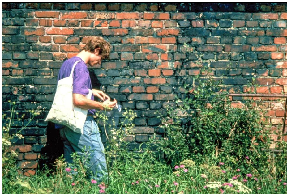
Figure 151: In contrast to Building 5a (see Figure 145, 167-169), the disinestation wing of Building 5b was used as a hydrogen cyanide delousing chamber for a longer period of time. Subsequently, the outside of its walls is covered with blue spots, unimpressed by 50 years of weathering here as well. Here the southern wall (August 1991, with the author).
