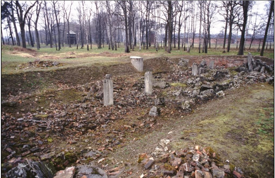
Figure 70: Morgue #1 of Crematorium III, with its roof utterly demolished (February 1997.).
