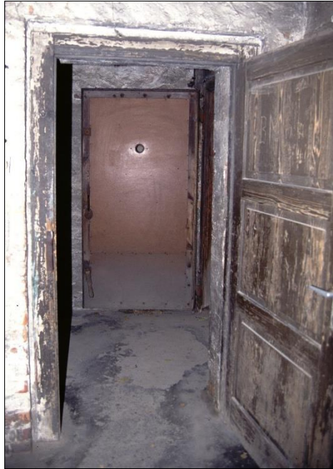
Figure 48: Look inside the air lock of the former SS air-raid shelter, with the open air-raid shelter door in the background.
