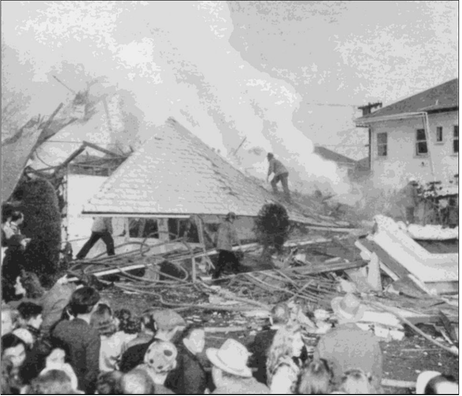
Figure 5: How not to get rid of termites: The concentration of hydrogen cyanide used was too high. One single spark, and the entire house blew up.
