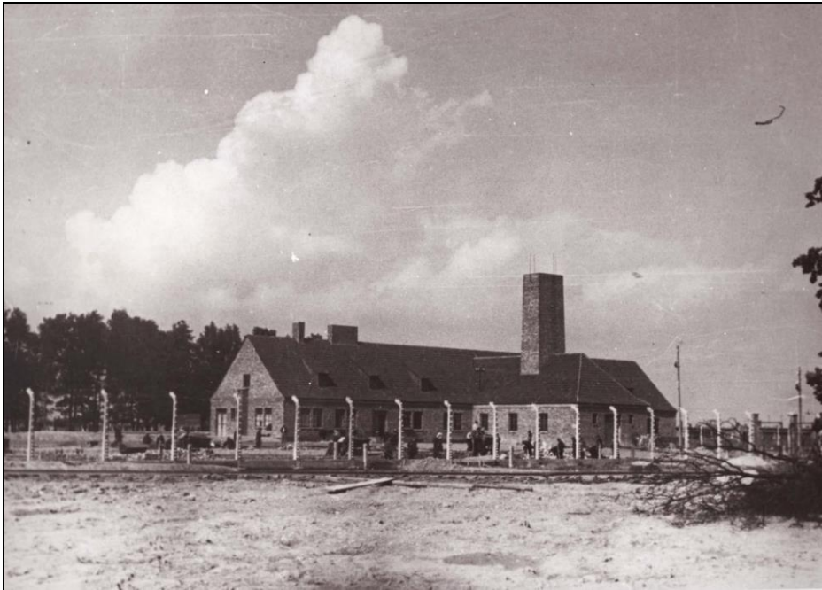
Figure 59: The finished Crematorium III. Photo taken in spring of 1943 by SS Unterscharführer Dietrich Kamann. Source: Yad Vashem Photo Archive, ref. 7741/4.
