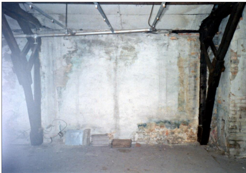
Figures 150a&b: Interior of the disinfestation wing of Building BW 5b, western part of the southern wall. The plaster, rich in lime, is only slightly stained. It has fallen off in certain areas. The mortar underneath is much more stained, see the close-up photo below. (© C. Mattogno, July 1992)
