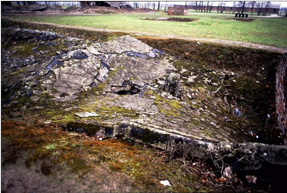
Figure 66: Morgue #1 of Crematorium II in Birkenau, collapsed roof, somewhat-intact rear section still accessible. Center: The last of the seven concrete pillars poking through the roof. A meter or so to the left: a hole chopped through the roof to gain access to the area below (see Figure 84, p. 139). (February 1997)
