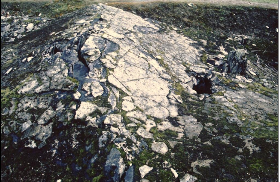
Figure 65a: Morgue #1 of Crematorium II in Birkenau, collapsed roof, somewhat intact rear section still accessible. Top right: The last of the seven concrete pillars poking through the roof. A meter or so to the left: a hole chiseled through the roof to gain access to the area below (see Figure 84, p. 139). (February 1997)
